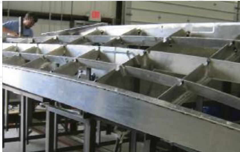
Aluminum Hull Frame Assembly Construction
